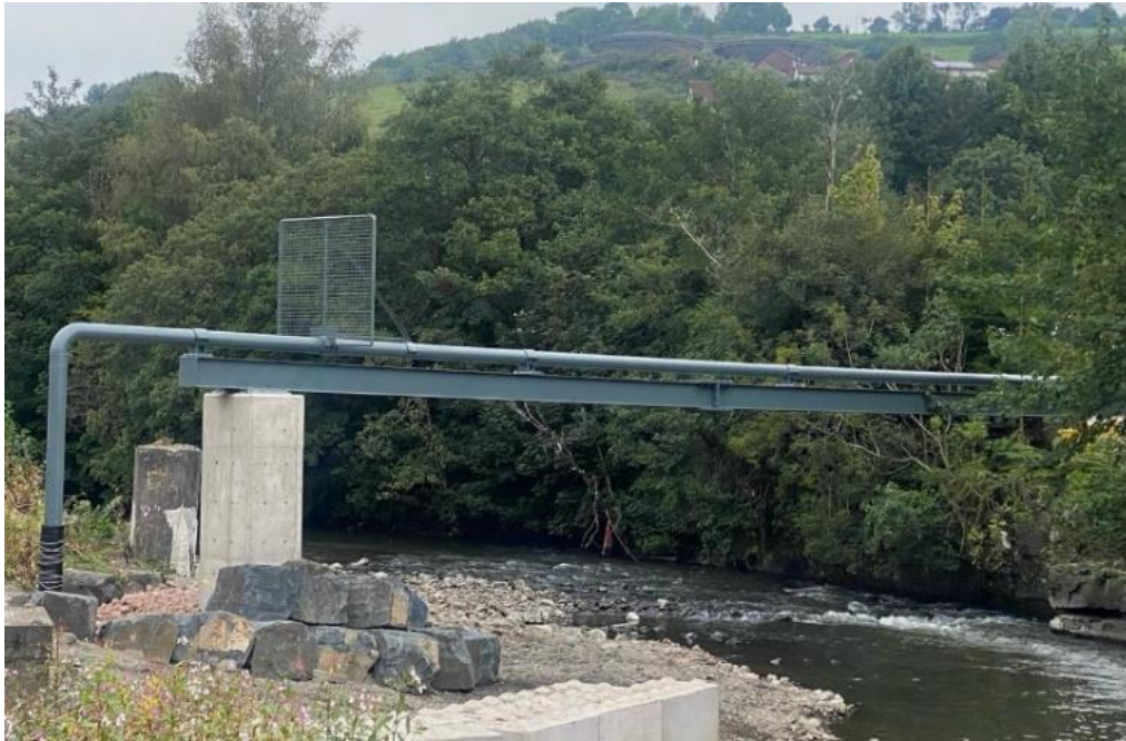
Fig. 2: Final diverted crossing above predicted flood height.
