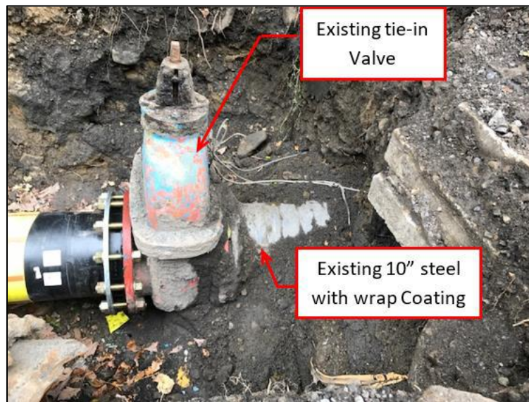
Figure 13 - New PE pipeline tying into existing valve
