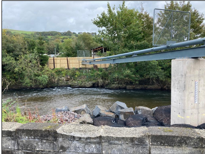
Figure 1 - Distribution steel pipeline crossing
