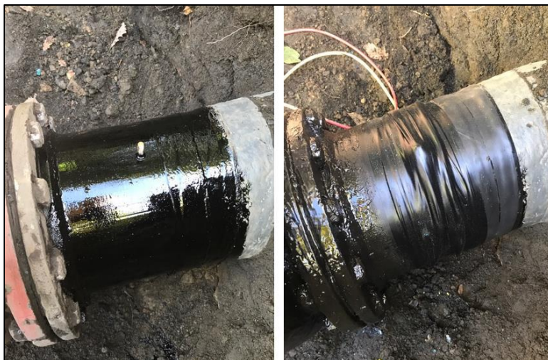
Figure 14 - Valve Flange Coated and Wrapped
