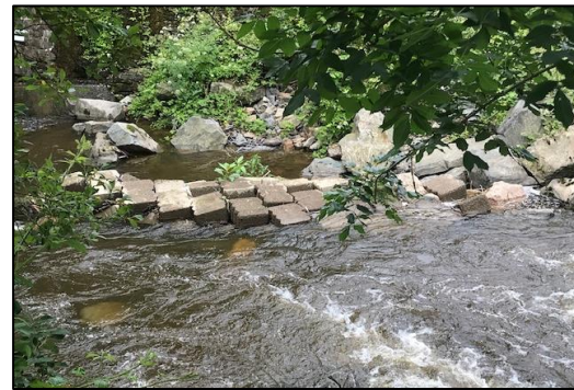
Figure 21 - Protective matting reinstated
