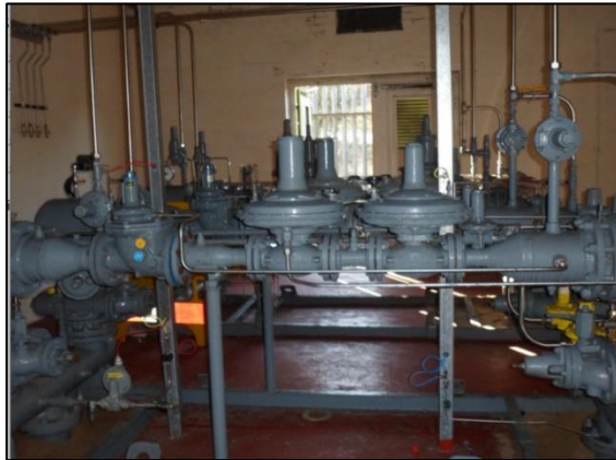
Figure 9 - Rhyd Y Blew IP-MP & IP-LP, before replacement
