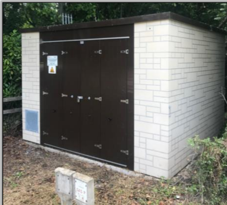
Figure 8 - Winchcombe Hospital District Governor, after new kiosk
